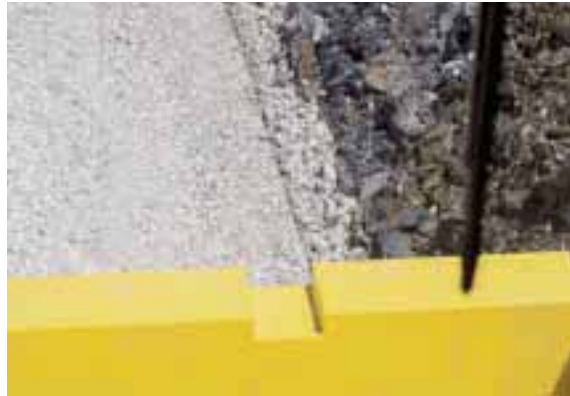
Precise compaction on edges with the optical track assistant.
